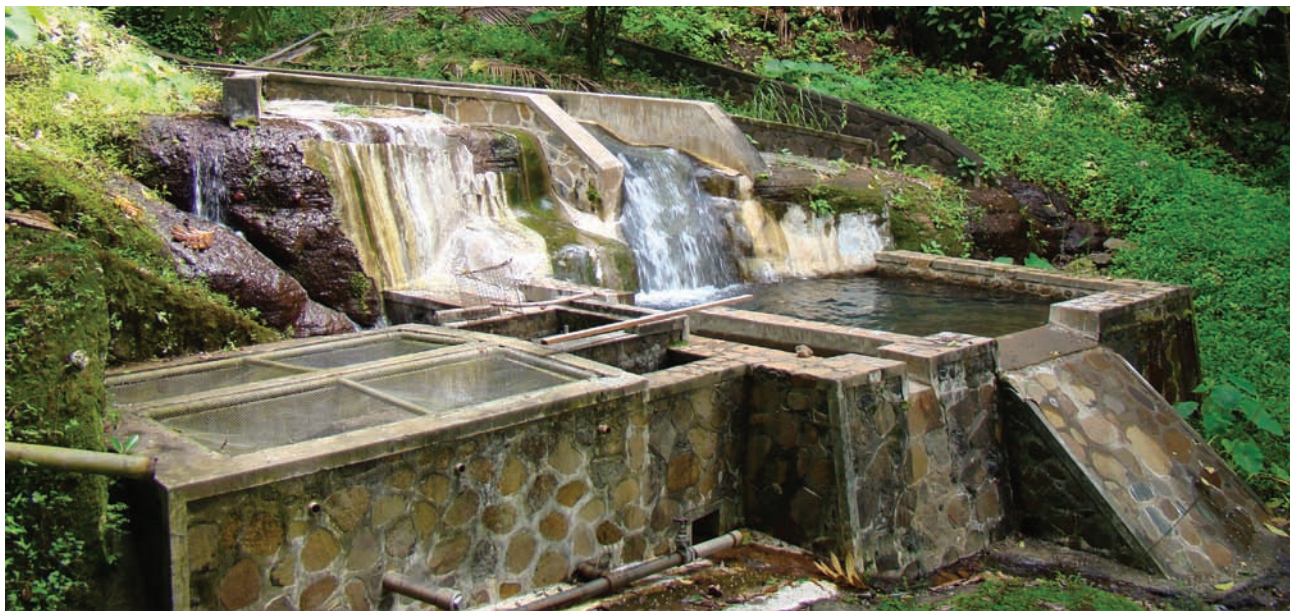
Photo 6.32 : Big Gut Water Catchment
