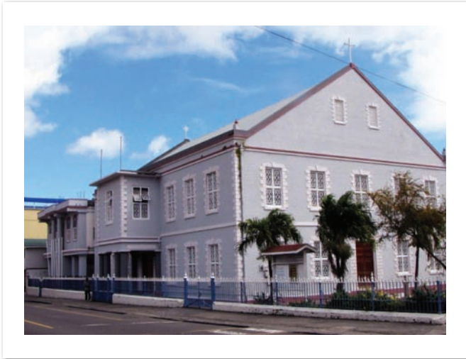
Photo 6.8: Kingstown Methodist Church: Constructed by Freed Slaves
