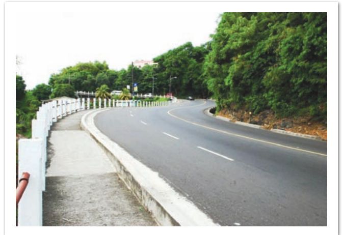
Photo 5.11: Road Network, Casson Hill
